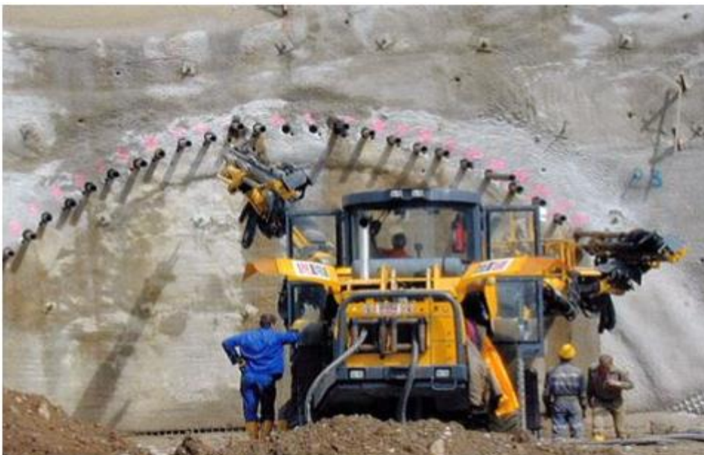
Figure 60. NATM support tubes installation (single Layer)
