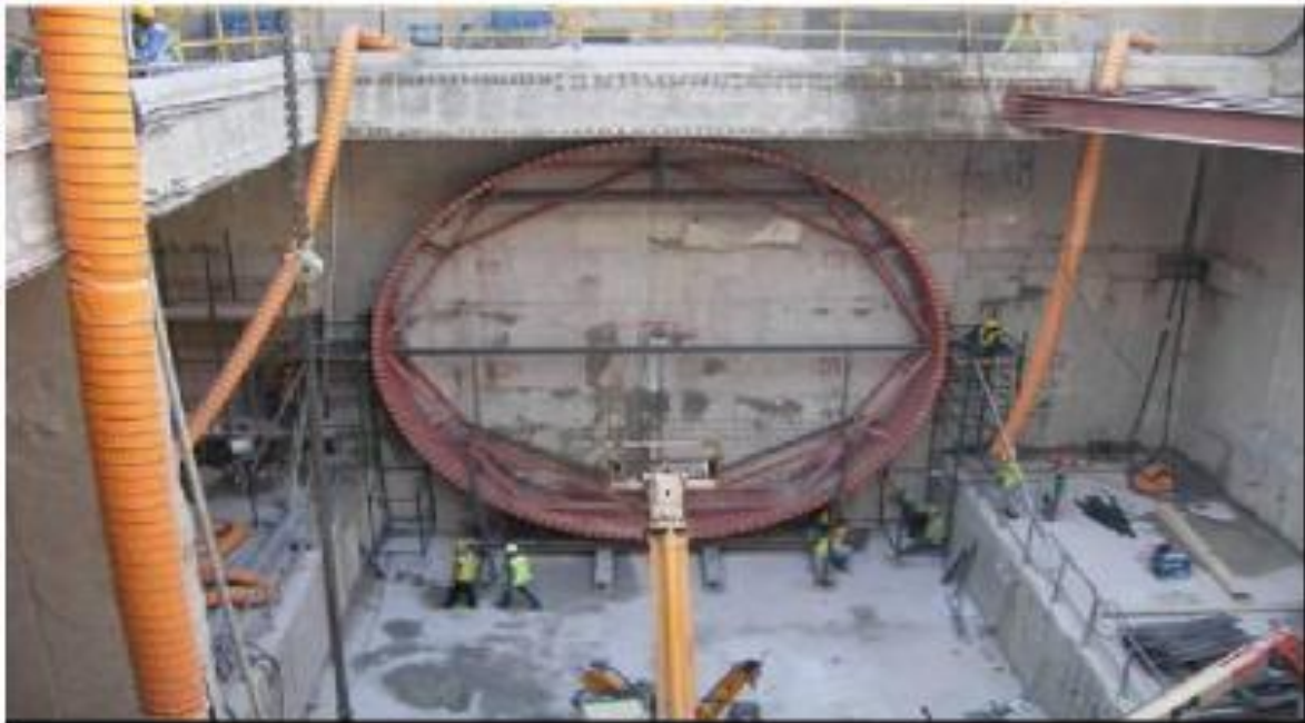
Figure 50. Launching Chamber
