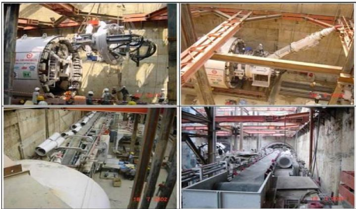
Figure 52. Erector, Screw Conveyor & Backup System
