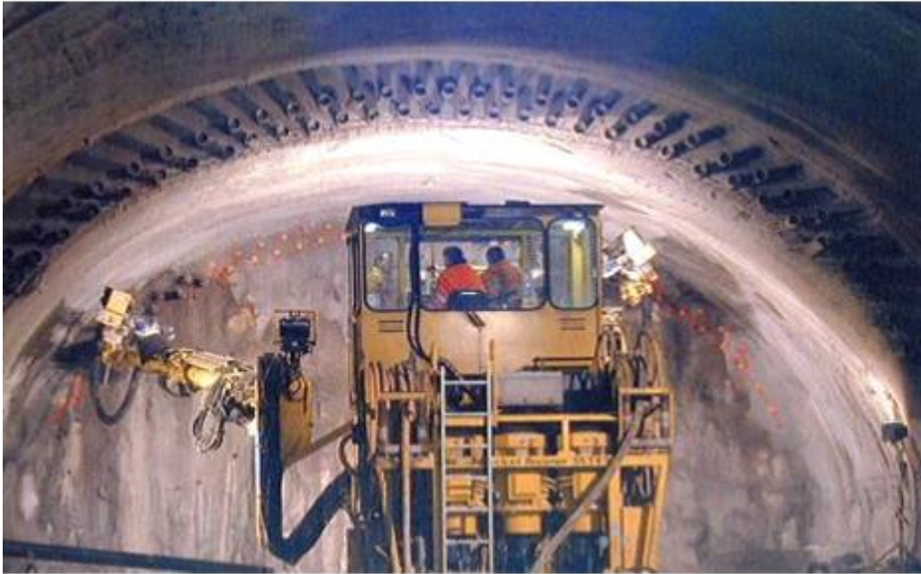
Figure 59. NATM support tubes installation (double Layer)
