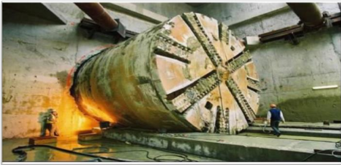
Figure 56. TBM Through the Diaphragm Wall
