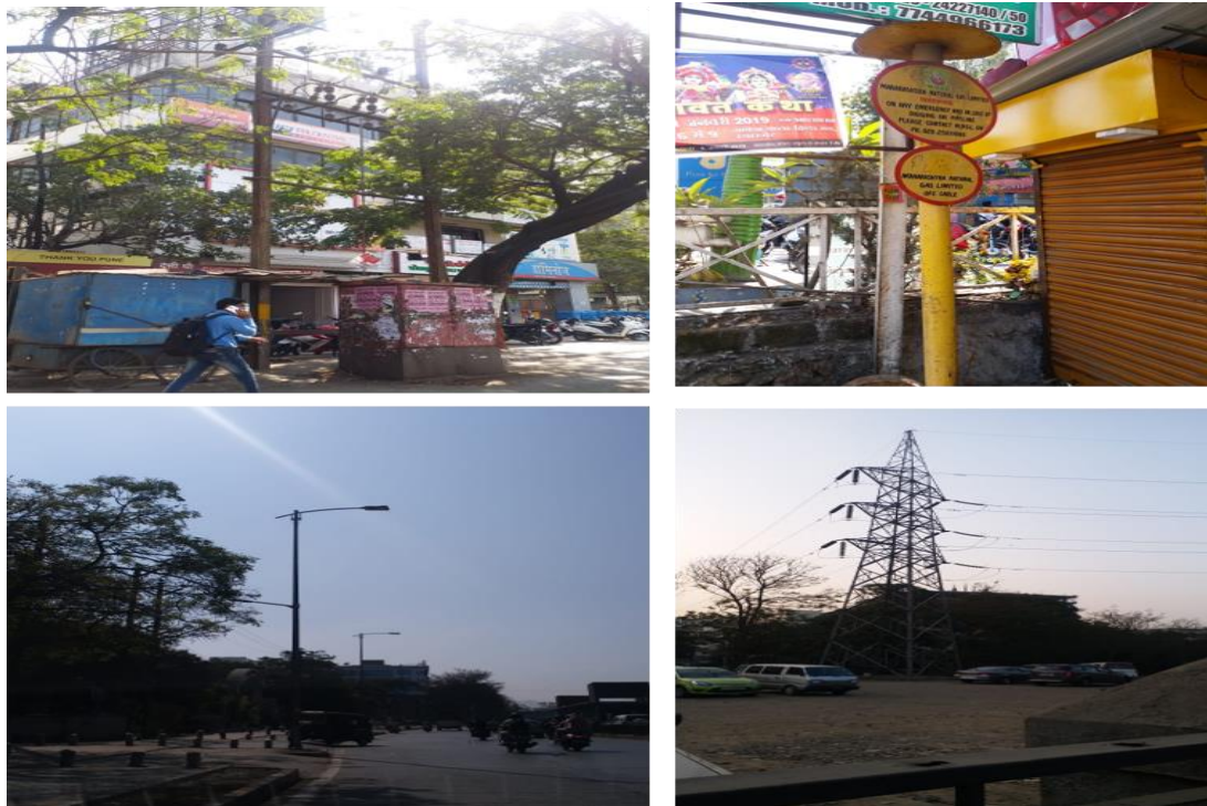
Figure 61. Affected Over ground utilities
