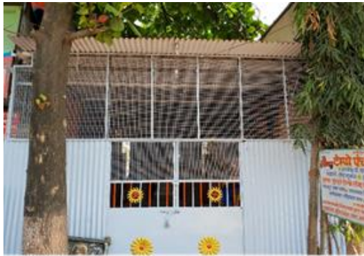
Saibaba Nagar Station Ch. 19.565
