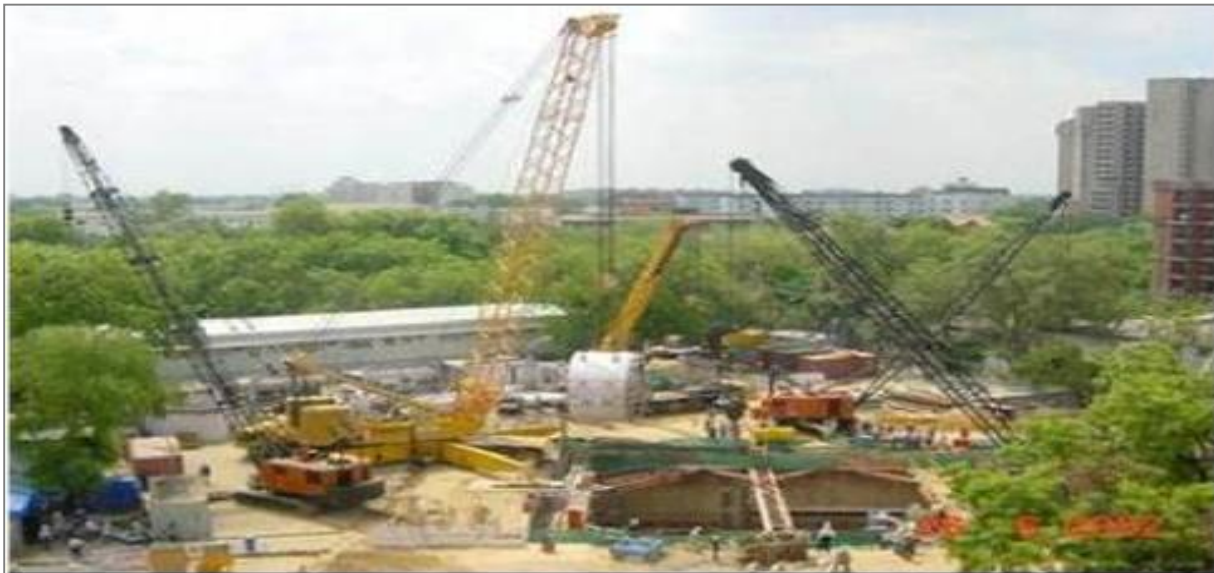
Figure 53. Main Shield Erection
