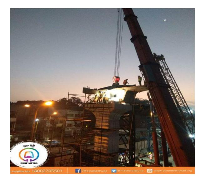
The segment has been built using Pre-Stressed Segmental Box Girder technology. The 45 ton segment was launched using 200 ton crane. There are normally 10 segments to complete a 28 meter girder. Once these segments are placed on `steel support', they are aligned and joined together with prestressing forces to act as a single unit.
